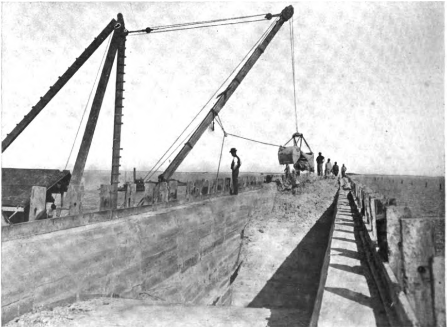
Long Key Viaduct.—Filling the last arch.
